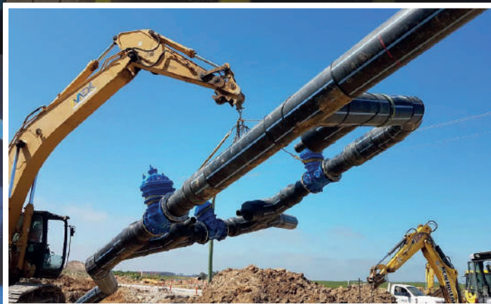
A bypass fabricated on site by PWS
